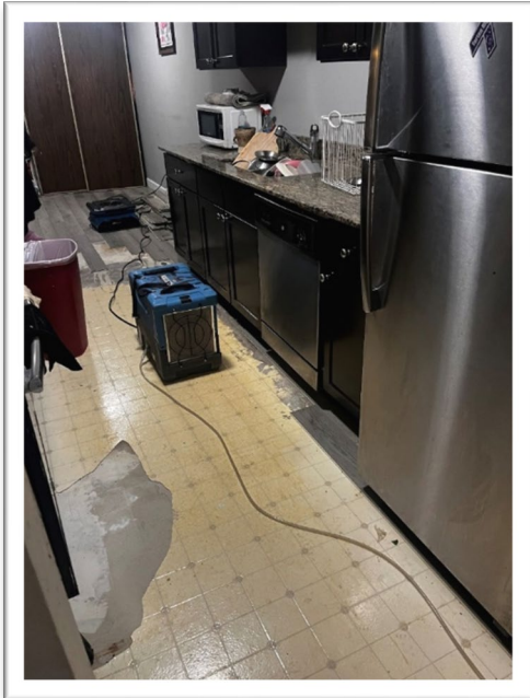
Above: Ripped faux tile vinyl flooring.
